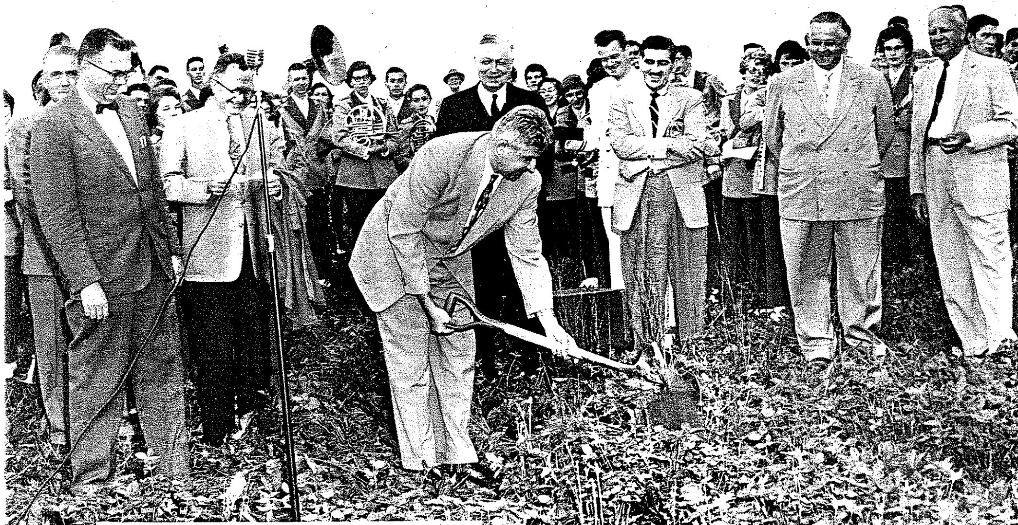
"Ground Breaking - May 24, 1956"
